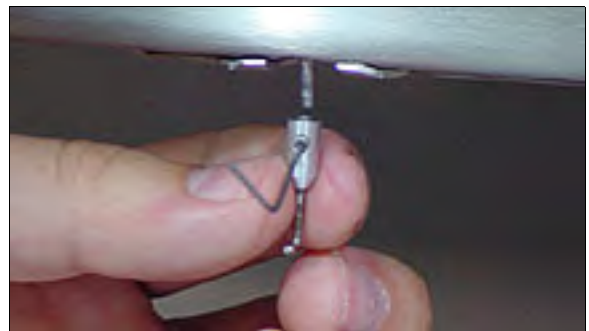
Installing wire pull hook
